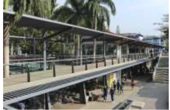
Figura 2.11: Bulevar USC Pampalinda
